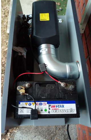
Picture 5. Installation on the box
